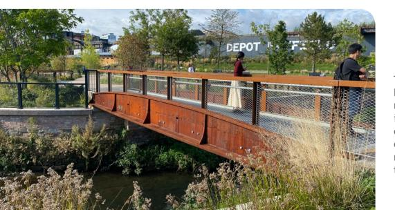
The design of Mayfield Park in Manchester has reused and upcycled many of the features that were on site, including the structure for the former culvert now used for the new footbridge constructions. Re-use of existing materials helped to reduce the cost of the park by £20 million.
